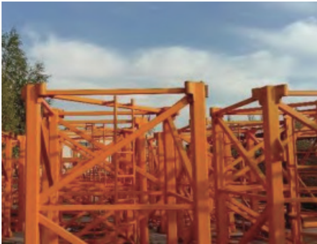
> 图3塔吊安装前构件检测
