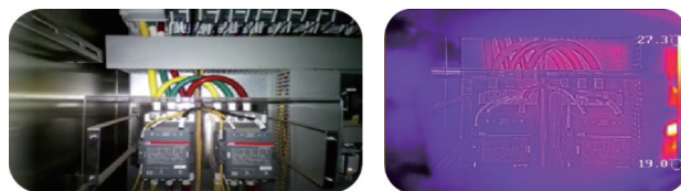
图7 断路器接头及红外效果 Fig.7 Circuit breaker connector and infrared effect
